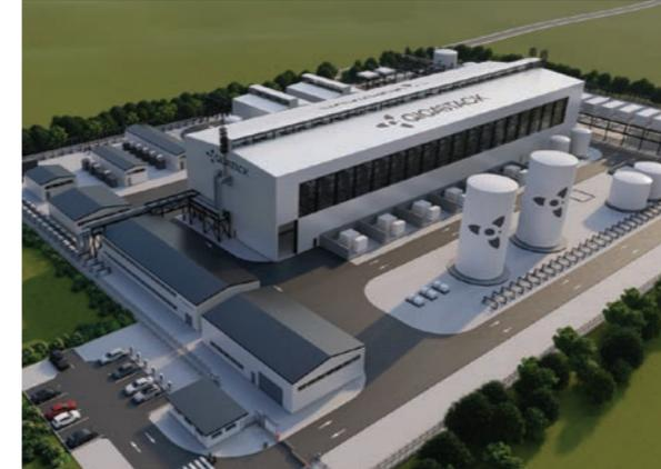
Gigastack is the UK's flagship green hydrogen project, led by a consortium of Phillips 66 Limited, Ørsted (UK) Limited, ITM Power (Trading) and Element Energy Limited. The project aims to harness offshore wind to power electrolysis and produce hydrogen, a low-emission fuel, to power industry.
